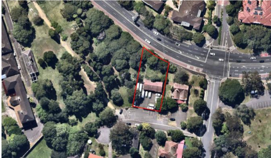
6 Victoria Road, Henley Part of Lot 880 DP 832717, North Sydney, NSW
