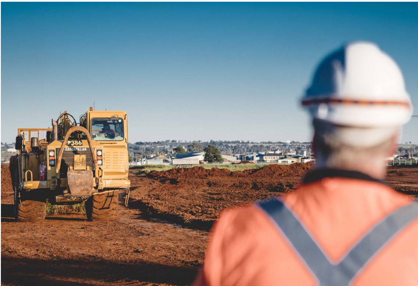
Road construction worker standing at a construction site near Dubbo
