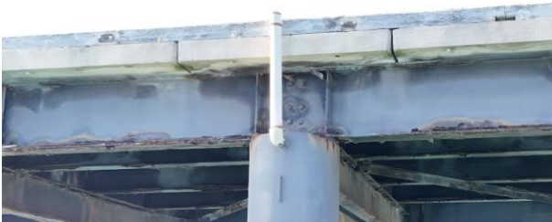
Photo 9 Example of Oil Filling Pipes at Top of CHS
