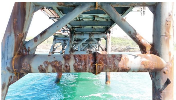
Photo 5 Example Photo of Bent Bracing
