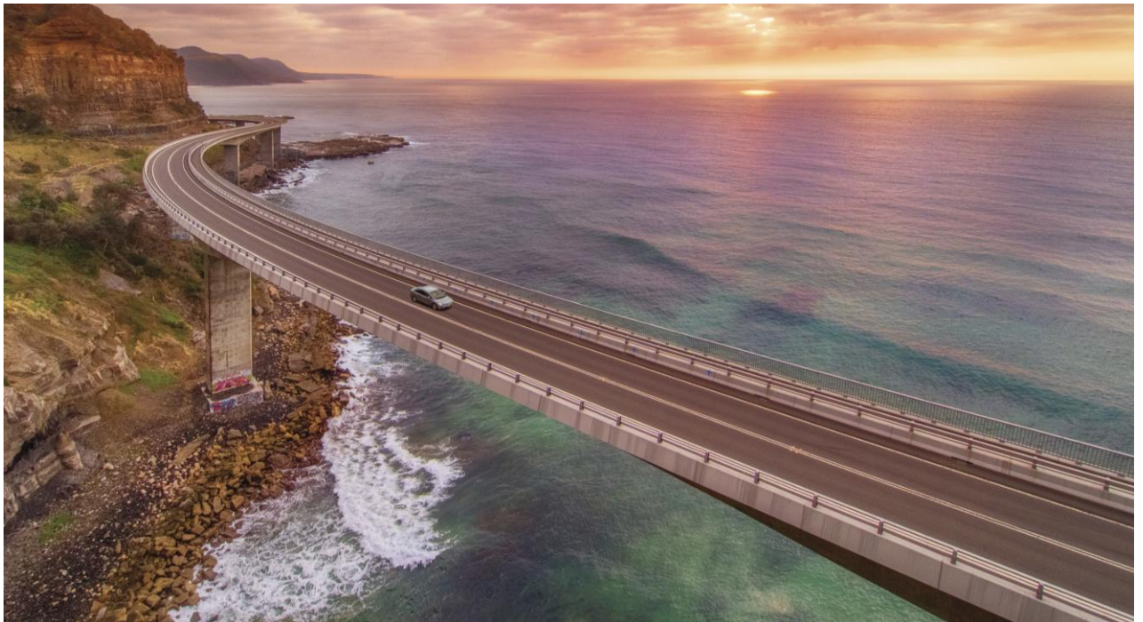
Seacliff Bridge © Destination NSW
