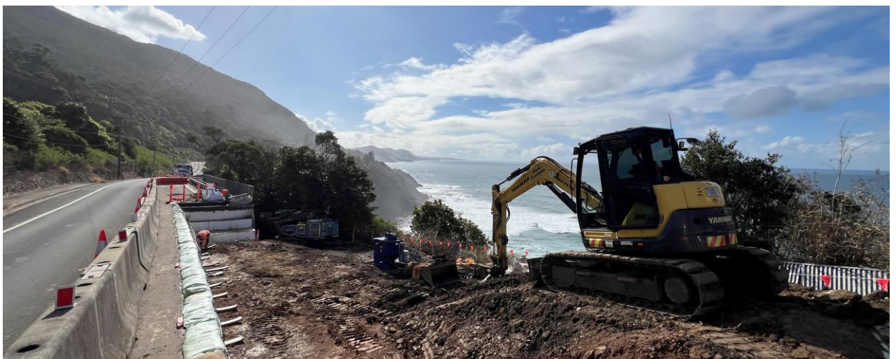
Slope repairs on Lawrence Hargrave Drive following damage in 2024
