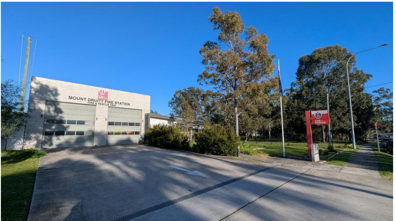
Figure 25 – The Mount Druitt Fire + Rescue Station to the east of the hospital on Railway Street
