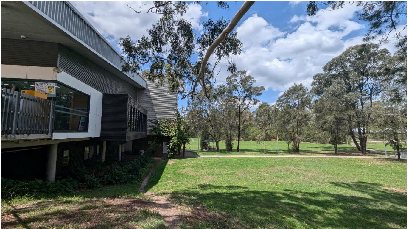
Figure 5 – Main Hospital Building to the left and the location of the proposed works / extension to the right.
