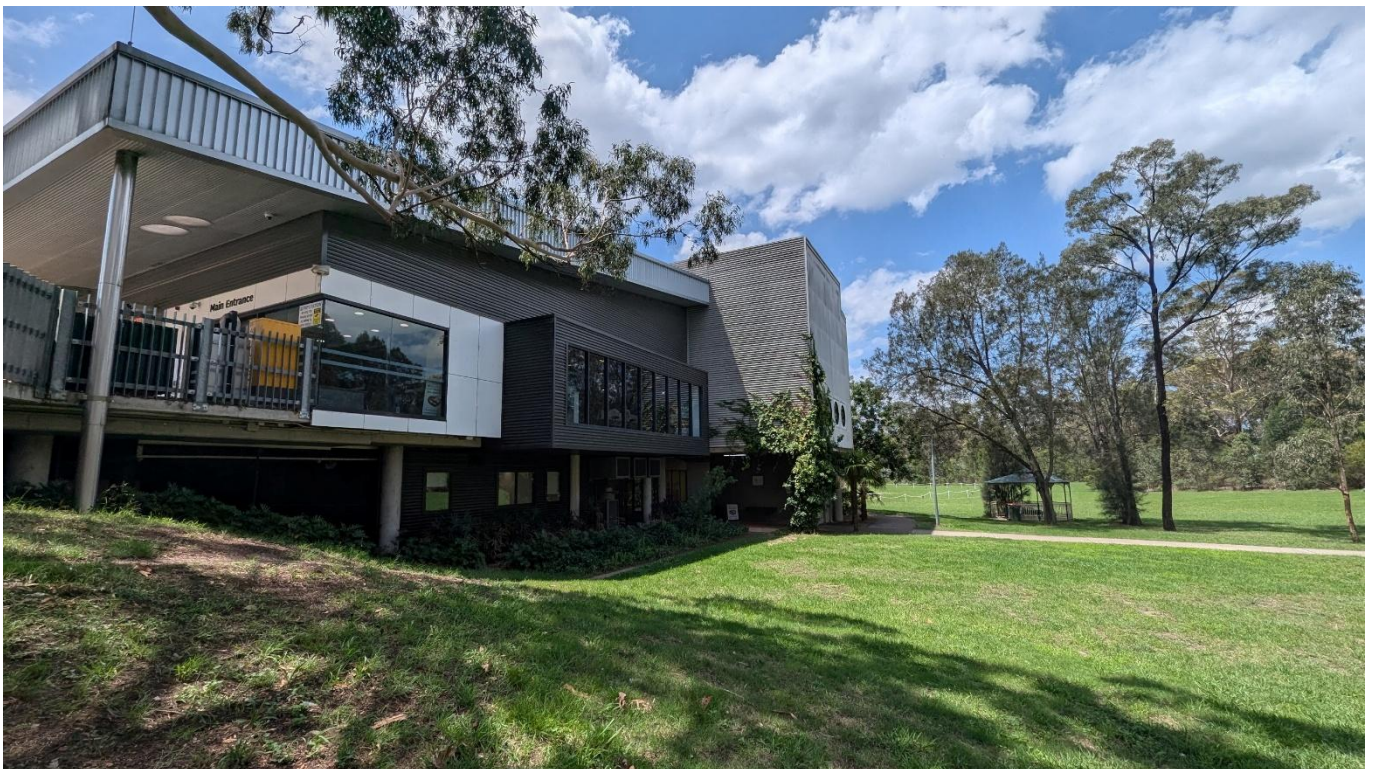
Figure 6 – Main Hospital Building to the left and the location of the proposed works / extension to the right.
