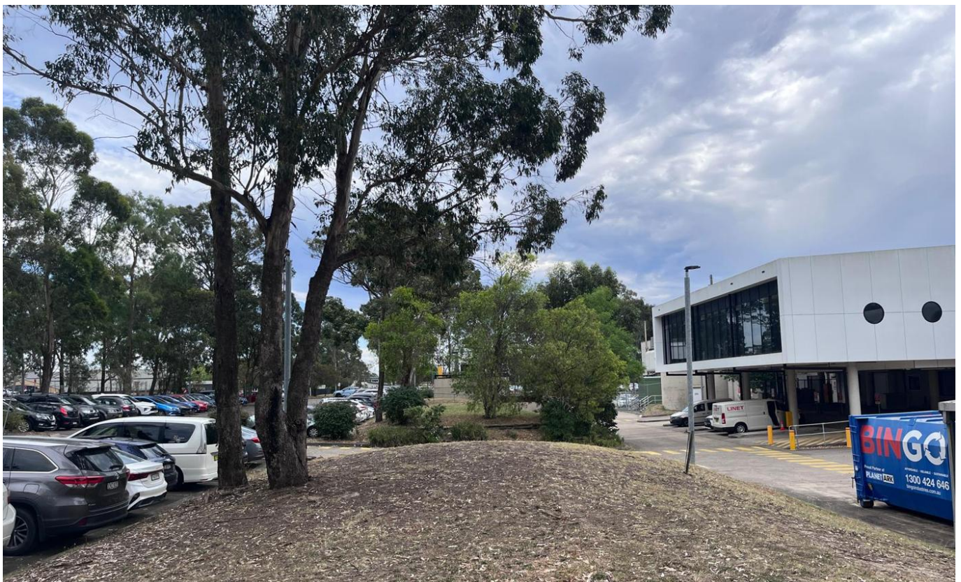
Figure 16 – Staff car park (P2) and loading dock area and location for part of new fire hydrant ring main
