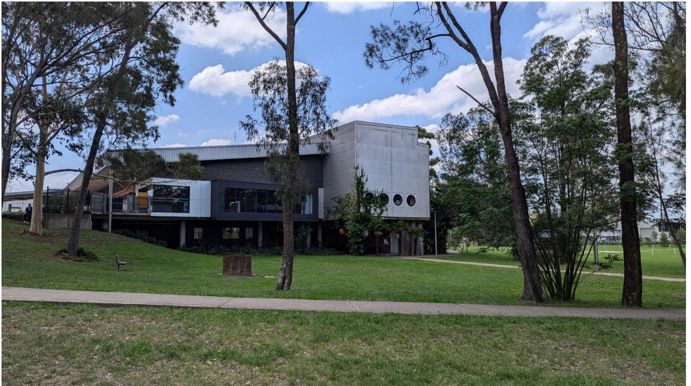
Figure 9 – Main Hospital Building and location of the proposed works / extension to the foreground and area subject to overland flows
