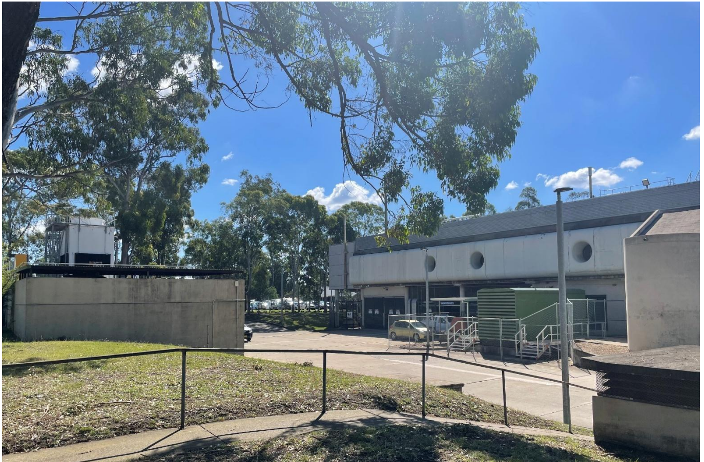
Figure 13 – Location of existing and new bulk oxygen plant and part of new fire hydrant ring main
