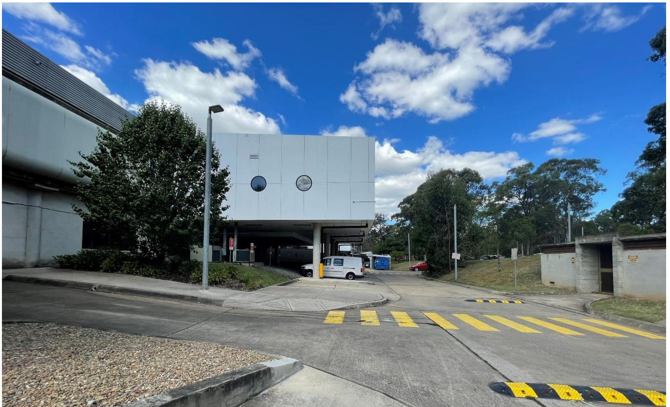
Figure 14 – Back of house and loading dock area and location for part of new fire hydrant ring main
