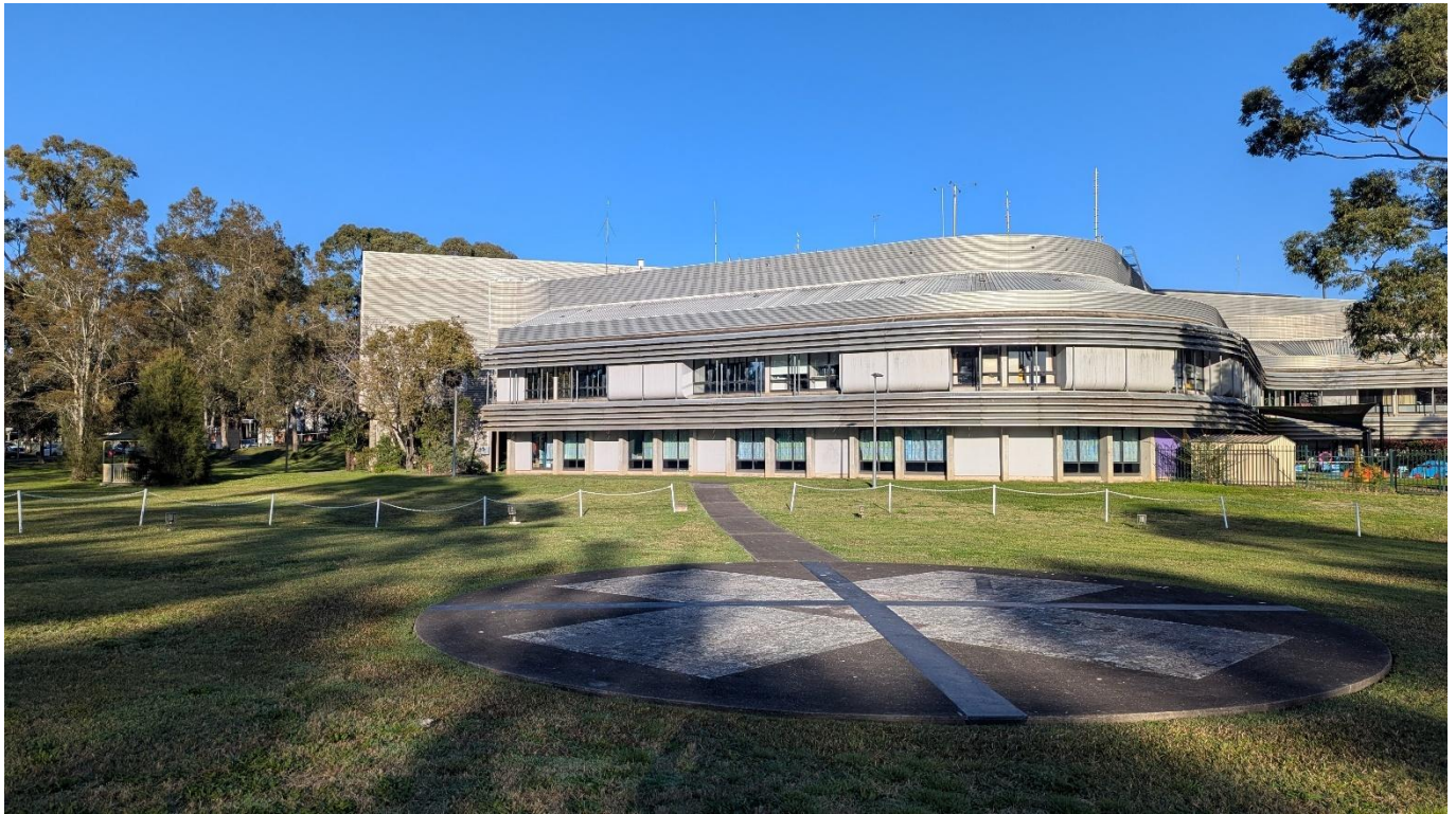
Figure 11 – Existing decommissioned helipad proposed for demolition with the location of proposed works / extension to the left
