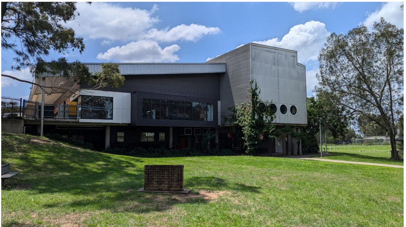
Figure 8 – Main Hospital Building and the location of the proposed works / extension to the foreground.
