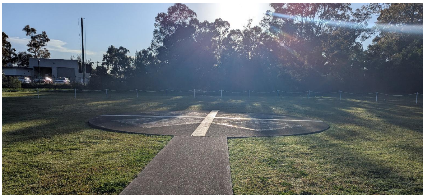
Figure 38 – Existing decommissioned helipad to be demolished
