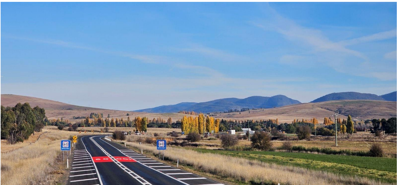
Figure 9. Town entry gateway treatments to improve road safety on the Monaro Highway at Bredbo
