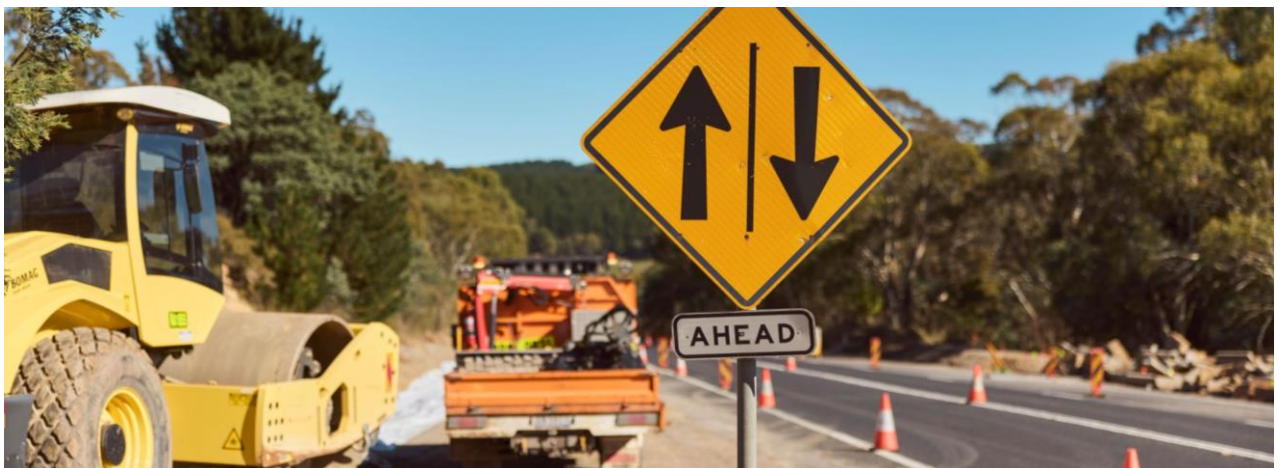
Figure 17. Road maintenance work being carried out
