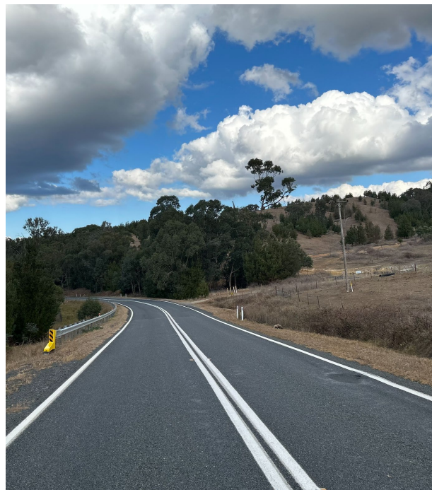
Road safety upgrade on Tumbarumba Road.
