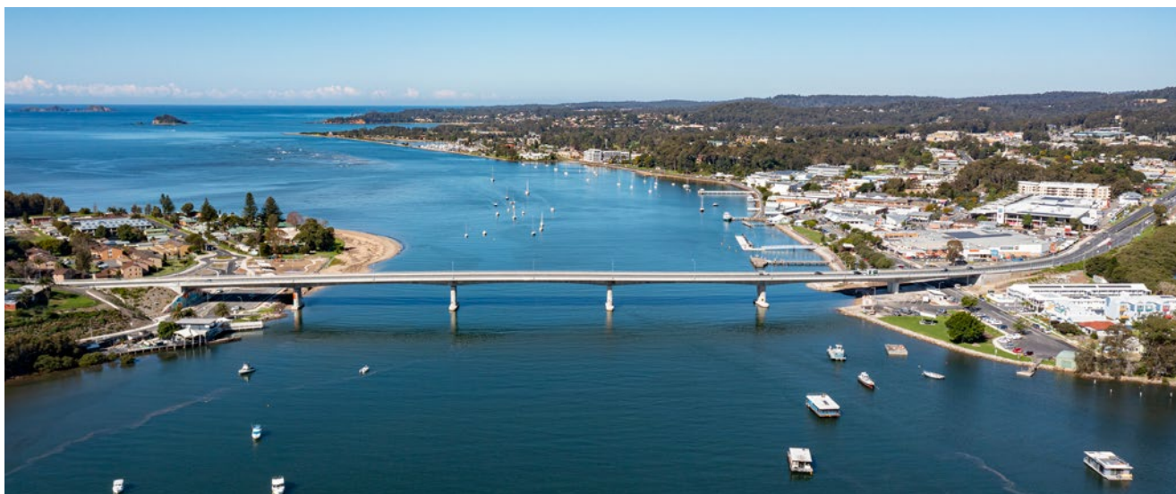
Aerial of Bateman's Bay Bridge over Bhundoo River / Clyde River at Bateman's Bay looking east
