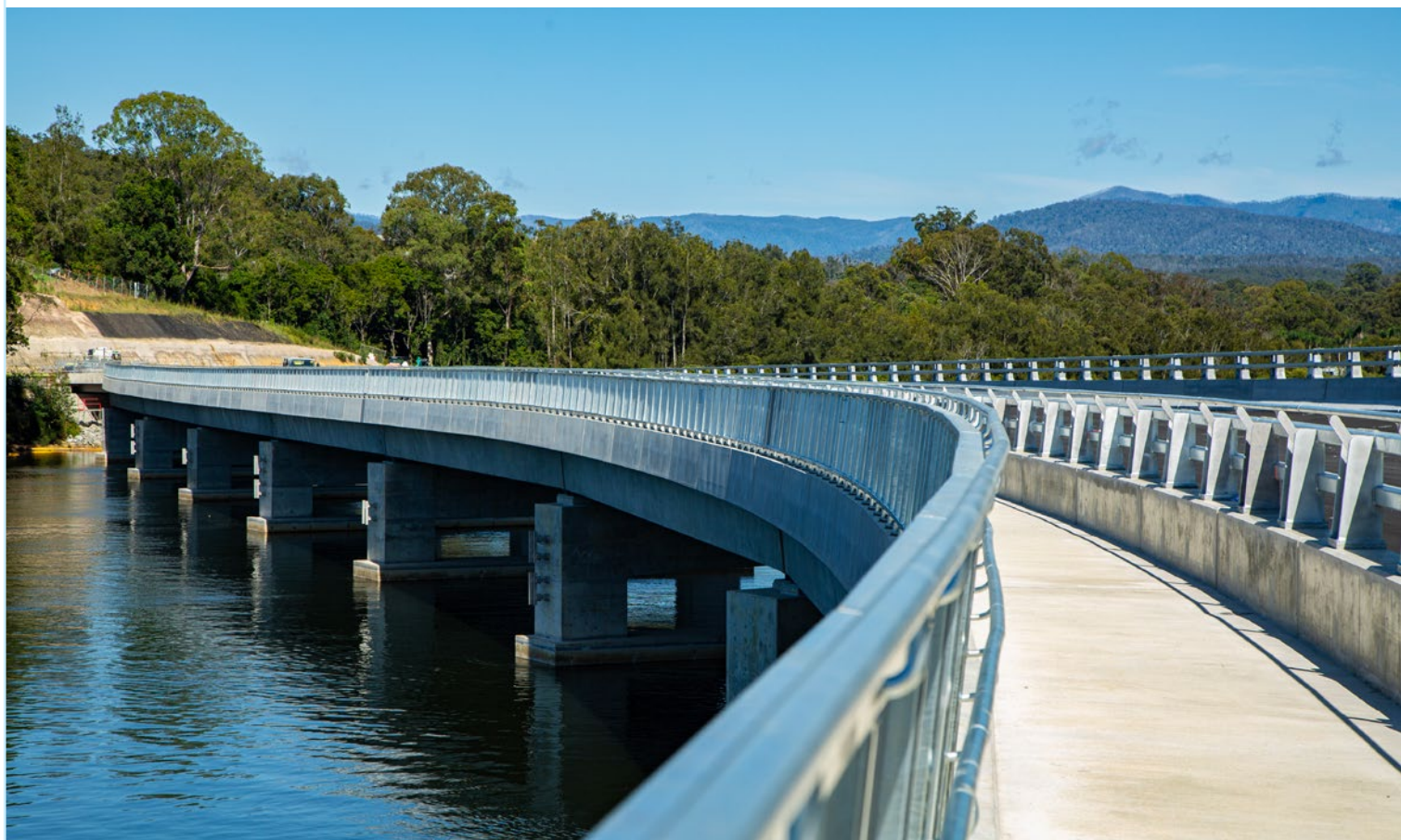
New Nelligen Bridge before opening to traffic
