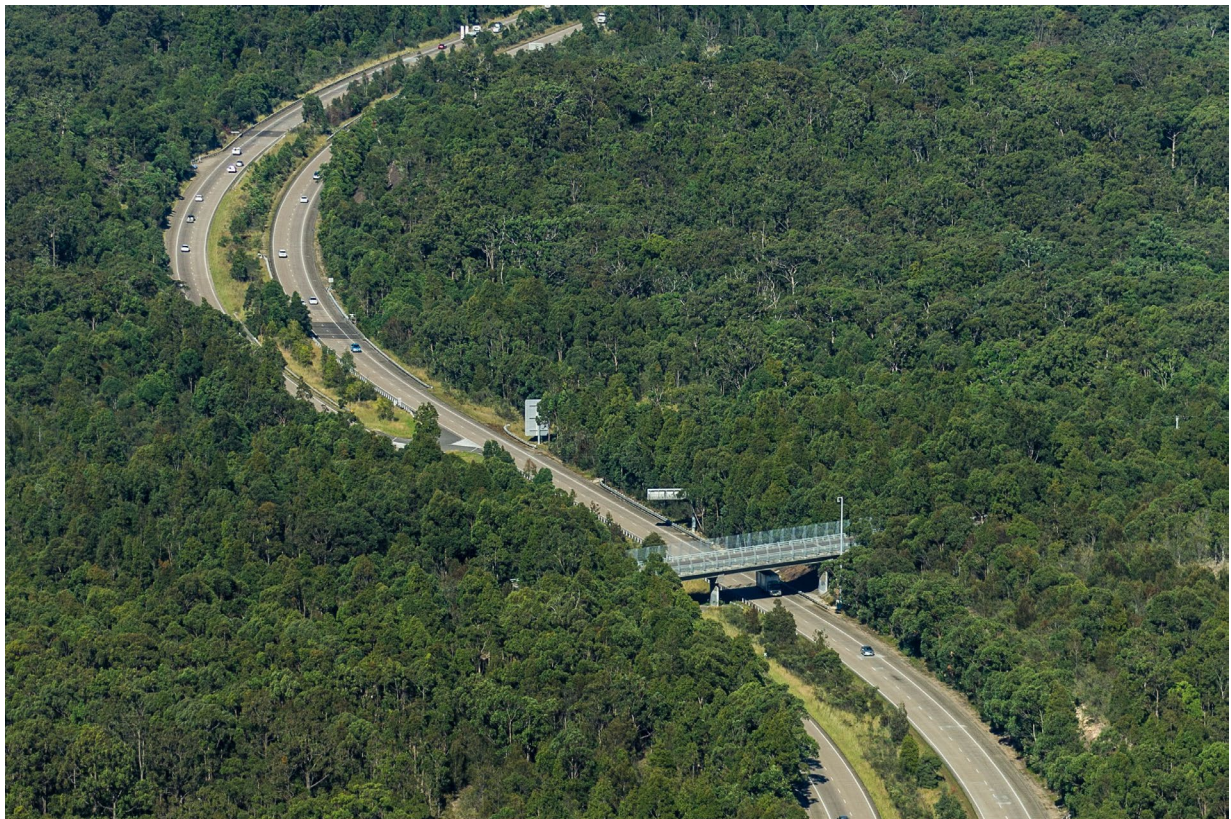
Figure 2. Aerial view of winding Pacific Motorway (M1) in Hunter Valley region.
