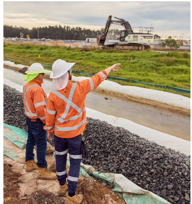
Figure 34. Field workers during construction of M1 Raymond Terrace extension.
