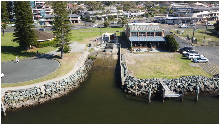
Aerial image of the slipway site where the new Tuncurry Boat Maintenance Facility will go.
