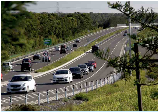
Newcastle Inner City Bypass upgrade
